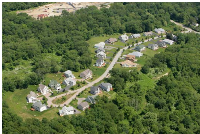
Figure 4.6– Alternative roadway design in Waterford, CT. Source: Tom Walsh, Shoreline Aerial Photography
