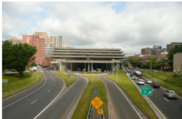
Figure 4.12 – Parking deck – New Haven,
