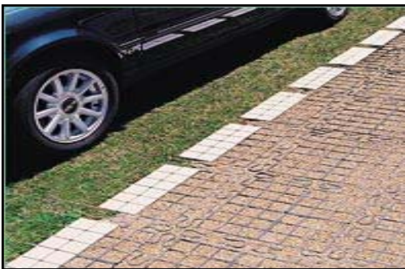
Figure 4.15 – Permeable pavement. Source: Connecticut, 2004.
