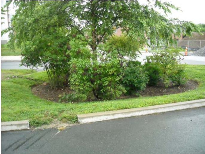
Figure 4.26 – Bioretention at University of Connecticut Storrs Campus –Mansfield. Source: Connecticut Department of Environmental Protection.
