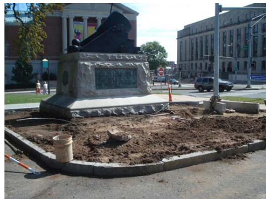
Figure 3.14 – Construction of a rain garden at Hartford Green Capitols Project. Source: Camp Dresser & McKee.
