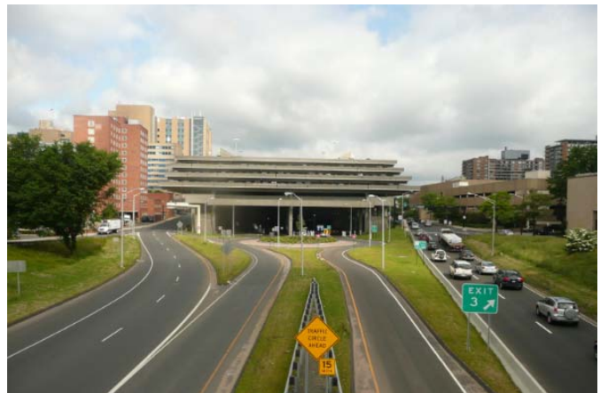
Figure 4.12 – Parking deck – New Haven,
