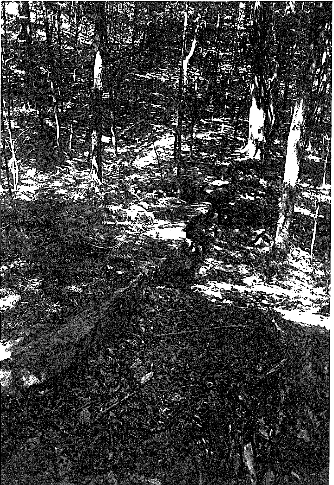
PHOTOGRAPH 2. MAIN DAM/RETAINING WALL. VIEW: WEST.
