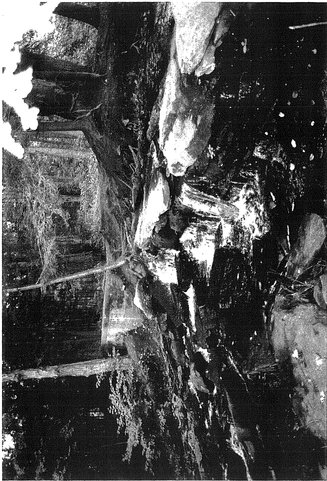
Headrace wall as currently overflowed by brook; concrete bulkhead in background; camera facing north photograph 7 of 10
