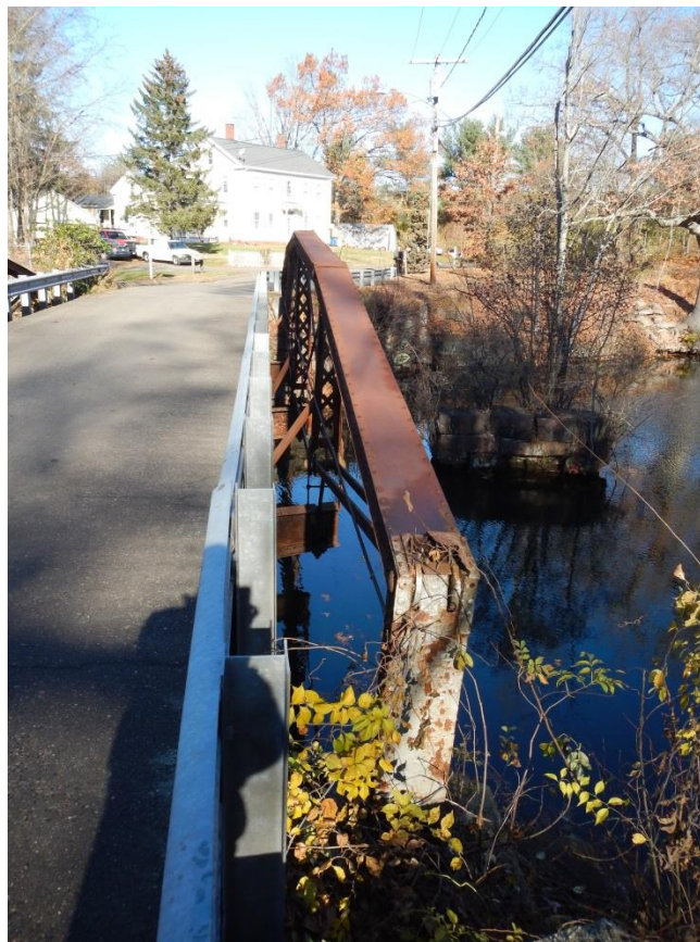
Image 2: The original truss supports its own weight on the brownstone abutments. The live load of the bridge is carried independently on a steel and concrete superstructure that was introduced in 1985. 11 Main Street is visible beyond the bridge.
