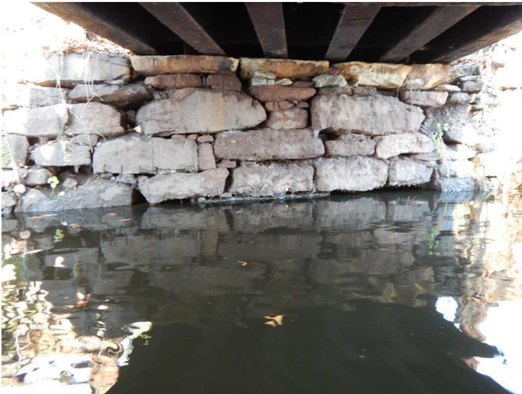
Image 4: North abutment of bridge. No mortar remains between the brownstone units and there are several voids in the abutment walls.
