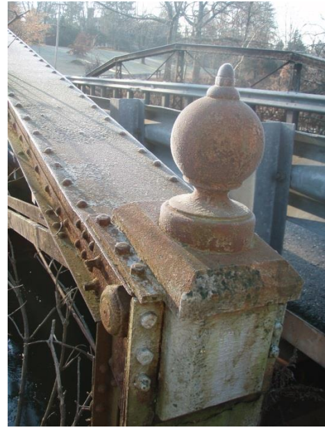
Image 3: Details of the lattice railing with cast iron rosettes and ball finial on Bridge #04575. These elements are original and distinctive of the Berlin Iron Bridge Company. Note that the grey gas line visible beneath the lattice railing will be relocated as part of this rehabilitation. It will no longer be visible within the replacement superstructure.
