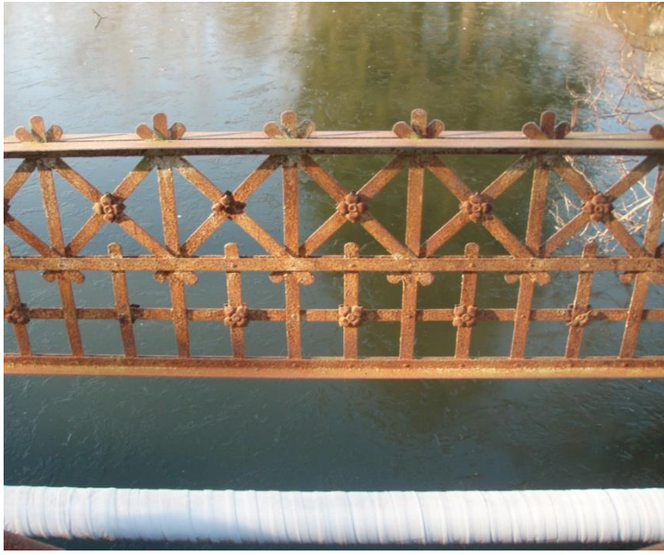
Image 3: Details of the lattice railing with cast iron rosettes and ball finial on Bridge #04575. These elements are original and distinctive of the Berlin Iron Bridge Company. Note that the grey gas line visible beneath the lattice railing will be relocated as part of this rehabilitation. It will no longer be visible within the replacement superstructure.
