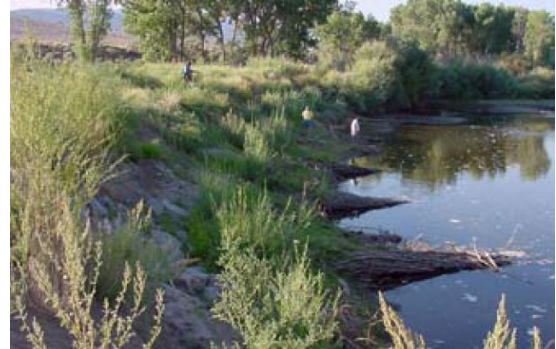
Bioengineering techniques used for slope stabilization and redirection (Source: NEH-654).
