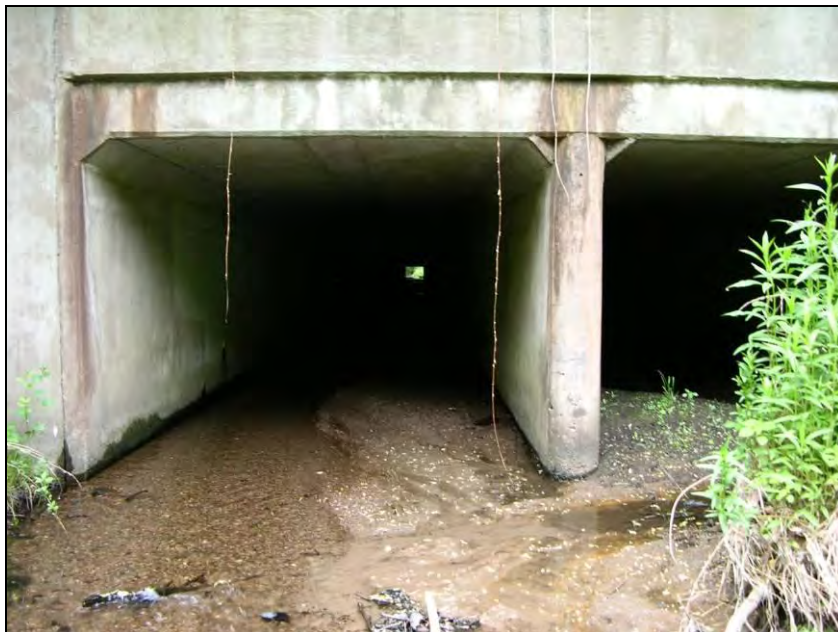
Twin box culvert along reach WR-05 underneath the onramp for I-84.
