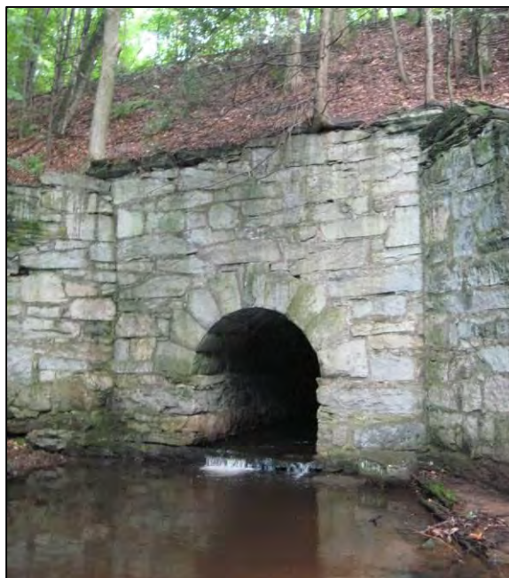
Arch-type railroad crossing (SC-02) constructed of stone and extending approximately 125 feet. The crossing may prevent fish passage and is suffering from downstream scour evidenced by the large pool shown in the photograph.
